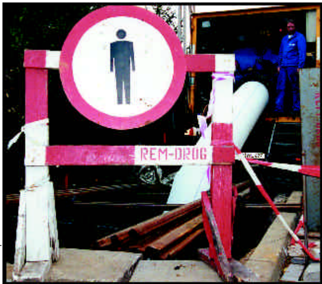
© Preuss Pipe Rehabilitation
