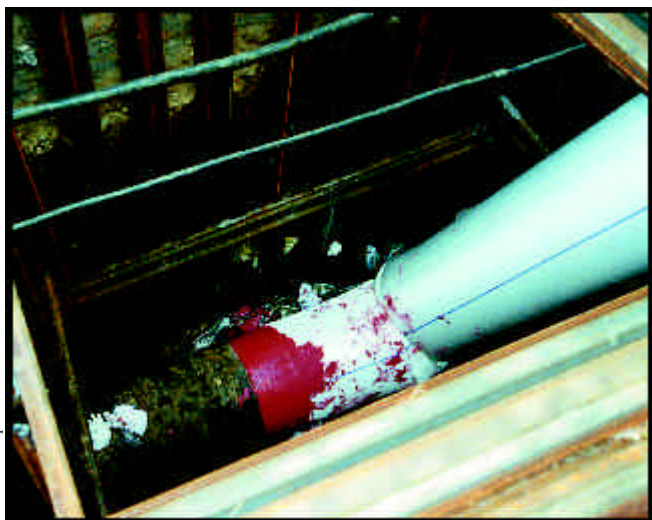
© Preuss Pipe Rehabilitation
